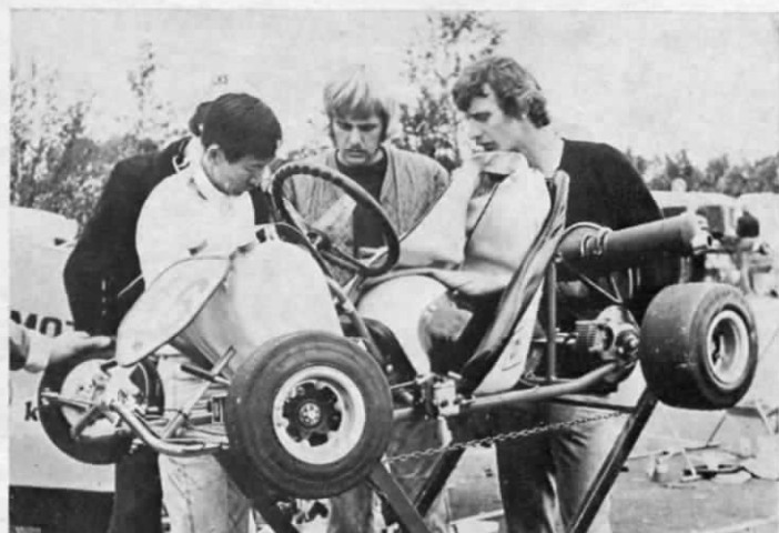
Probably the most unconventional kart at the Championships, to European eyes at any rate, was the American Margay Cheetah of Hong Kong's Harold Lee. It was equipped with four-wheel hydraulic brakes and twin distinctive looking fuel tanks apparently identical to those once familiar on Fox karts.
